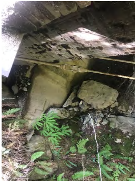
Left Bank Abutment when facing downstream
