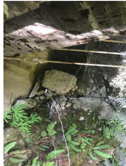
Left Bank Abutment when facing downstream
