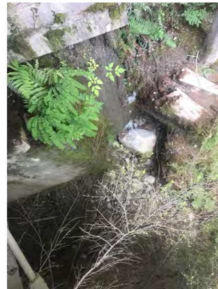
Left Bank Abutment when facing downstream
