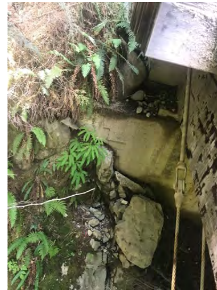
Left Bank Abutment when facing downstream
