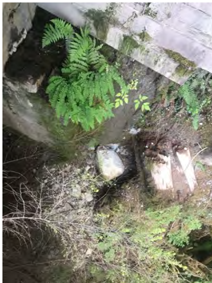
Left Bank Abutment when facing downstream
